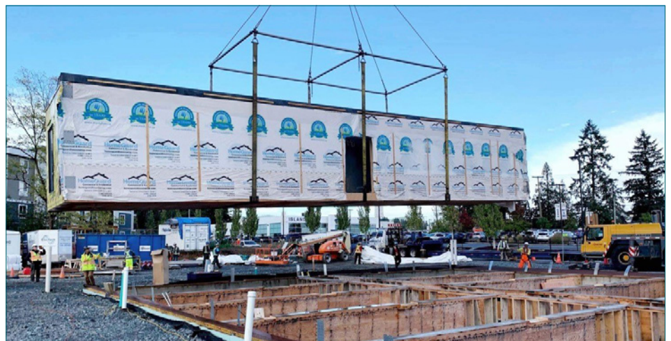
Sq'umul' Shelh Lelum' in North Cowichan, under construction.
