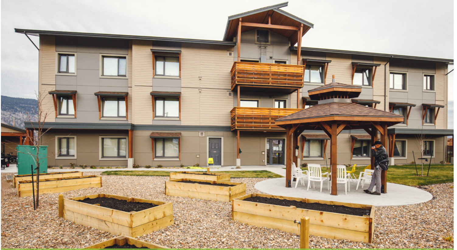
Juniper House in Merritt, certified to the International Passive House standard.
