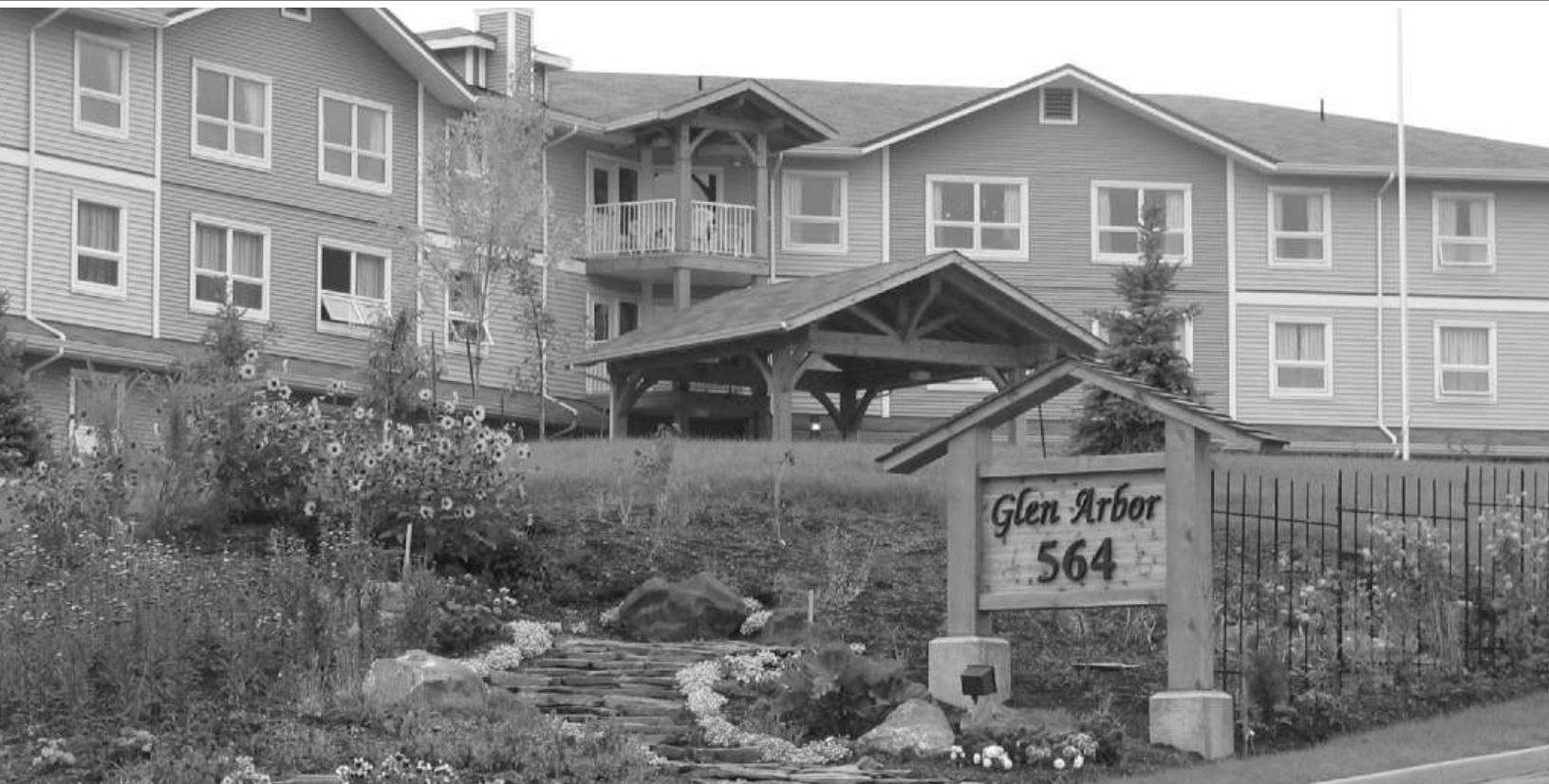
Glen Arbor — 34 supportive seniors' housing units in Williams Lake operated by the Cariboo Park Home Society and developed in partnership with BC Housing, Canada Mortgage and Housing Corporation (CMHC), City of Williams Lake and other donors.
