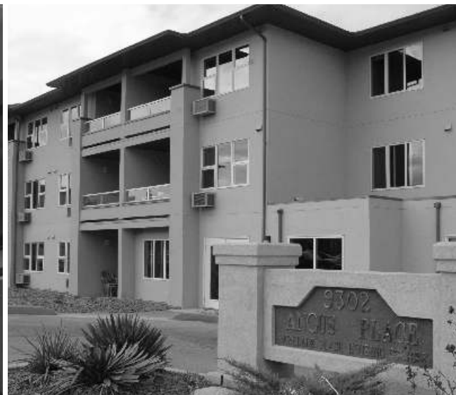
Angus Place — 33 units of supportive seniors' housing operated by Parkdale Place Housing Society in Summerland and developed in partnership with BC Housing, CMHC and District of Summerland.
