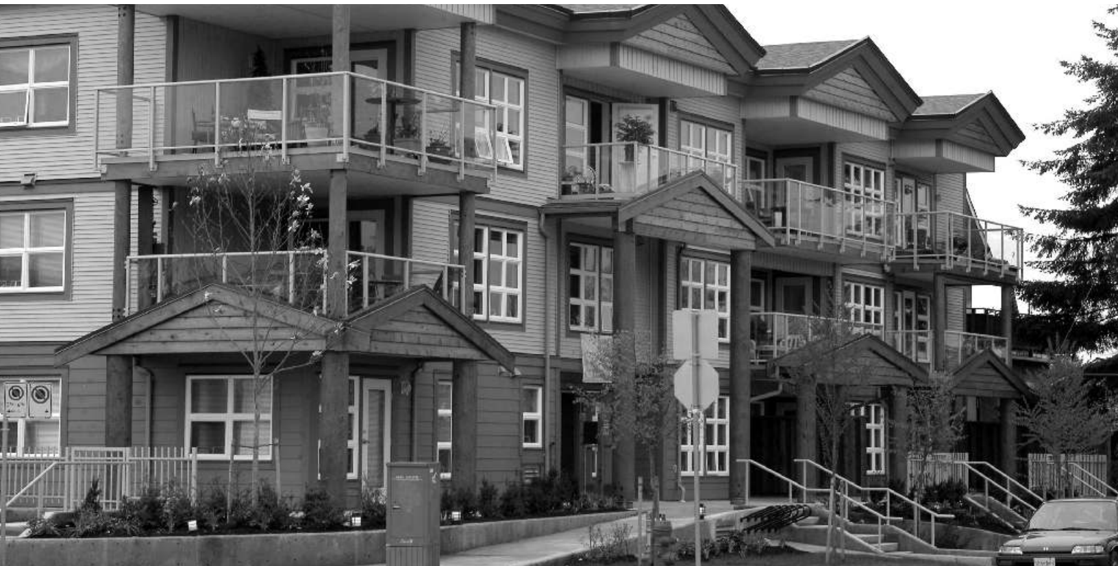
Lu'ma Native Housing's Aboriginal Patients' Lodge in Vancouver developed in partnership with CMHC, BC Housing, City of Vancouver and other funders.
